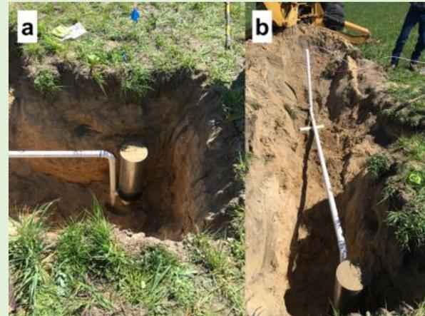
Figure 1. Drain gauge installation showing depth below soil surface (a) and the 2-inch PVC access pipe for the sample tube and pressure transducer cable (b).
